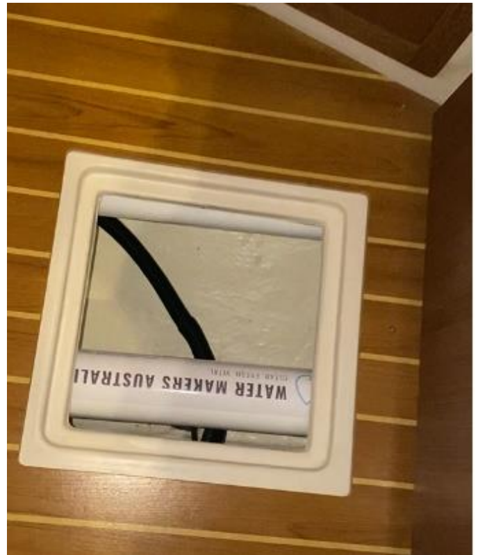
RO Tubes under floor outside forward head
